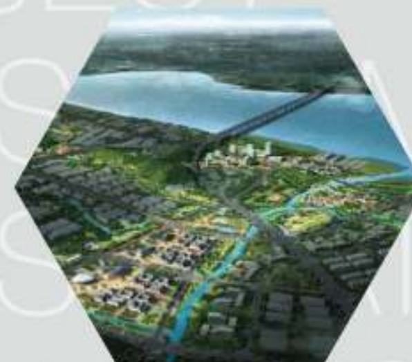
台州市椒江区绿色药都特色小镇建设项目 Construction Project of Green Medicine Characteristic Town in Taizhou (Jiaying)
