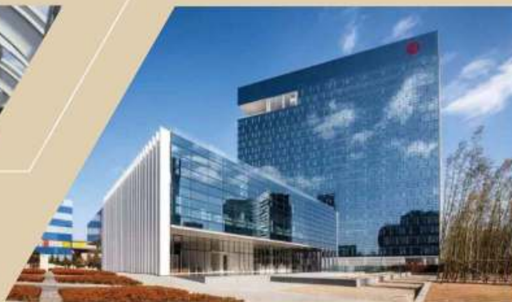
中国银行金融大厦 Financial Building of BOC
