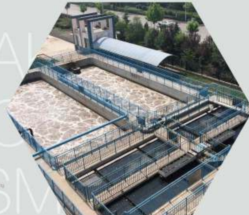
扬州市第三污水处理厂项目 The Third Sewage Treatment Plant in Yangzhou
