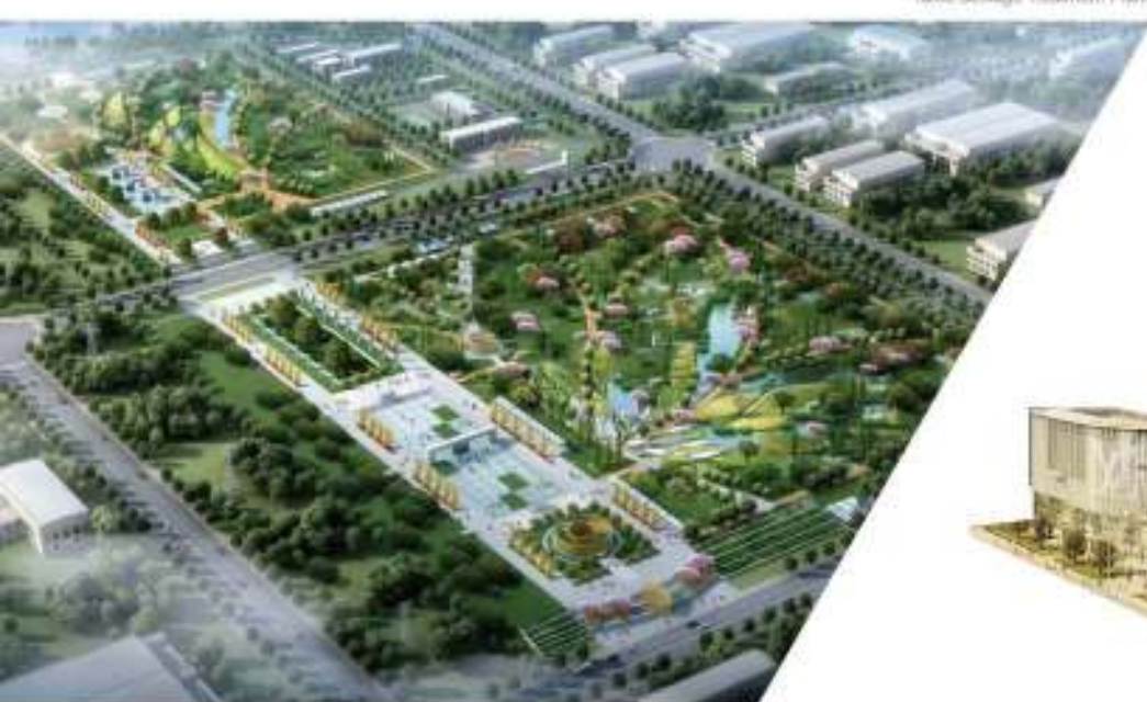
泰和污水厂 Tahe Sewage Treatment Plant
