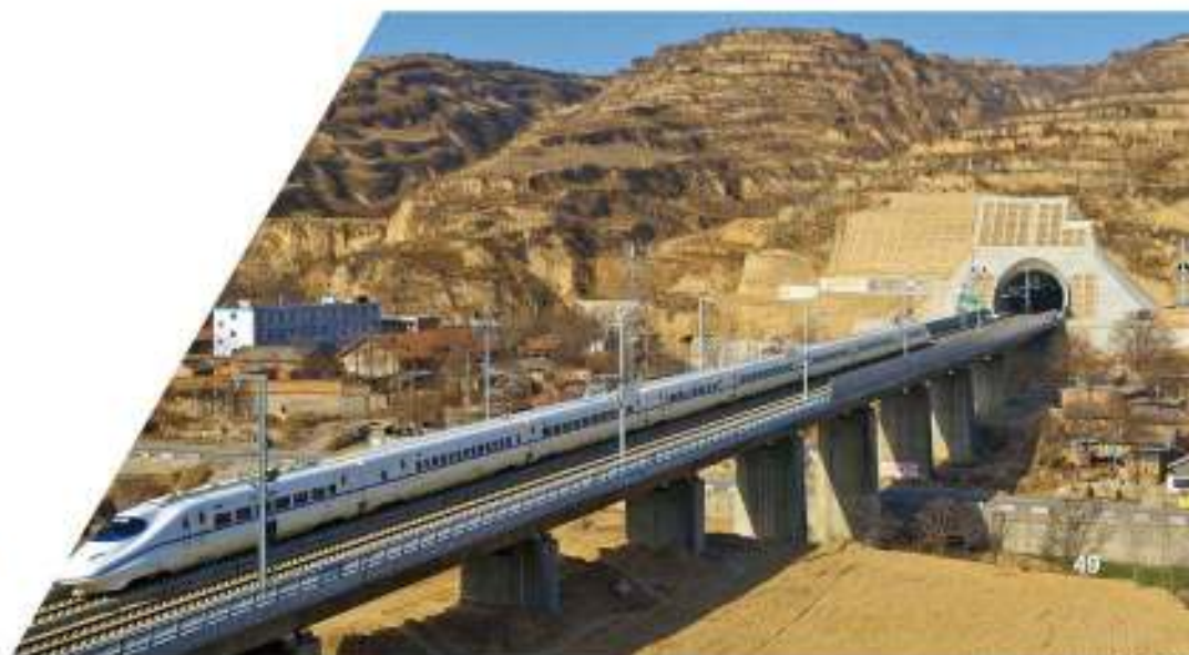
上海铁路局下穿铁路工程系列 Series of Underpass Railway Construction Projects of Shanghai Railway Bureau
